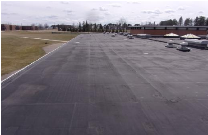
Photo 7 Wylie Elementary School February 2023 Area C: Overview
