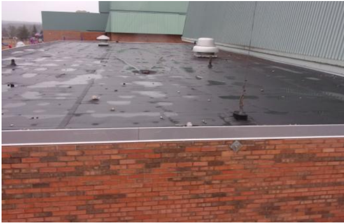
Photo 21 Wylie Elementary School February 2023
