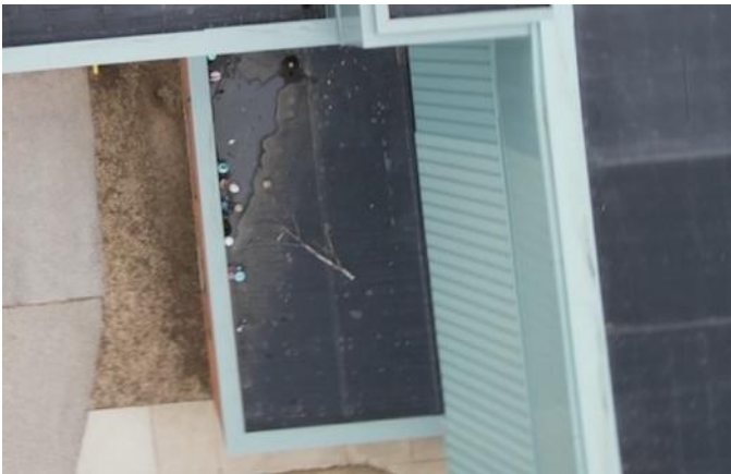
Photo 31 Wylie Elementary School February 2023
