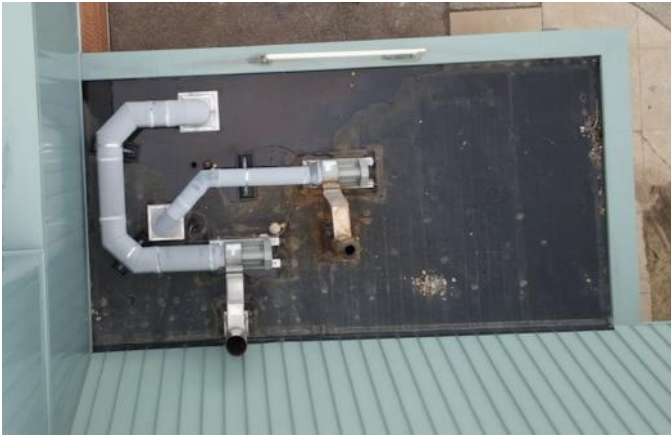
Photo 34 Wylie Elementary School February 2023
