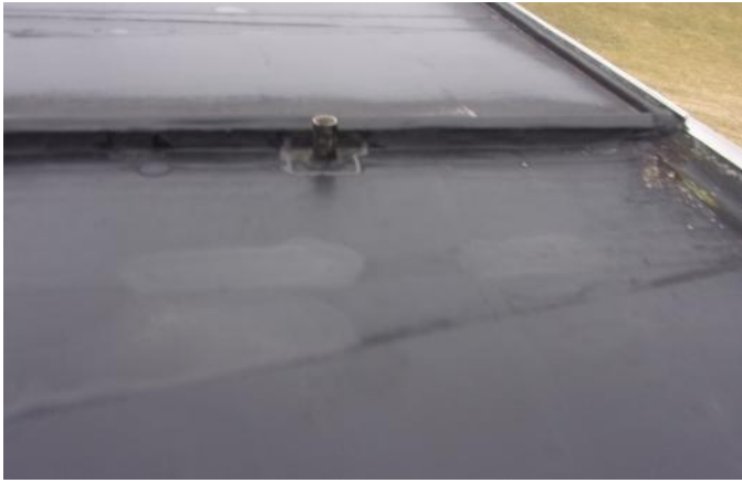
Photo 17 Wylie Elementary School February 2023
