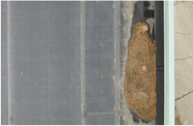
Photo 33 Wylie Elementary School February 2023
