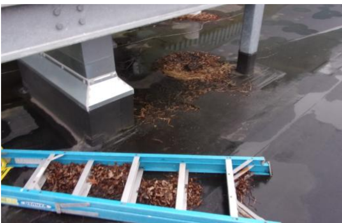
Photo 24 Wylie Elementary School February 2023
