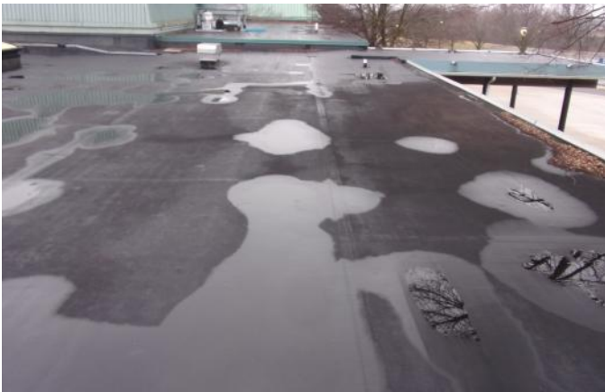
Photo 19 Wylie Elementary School February 2023
