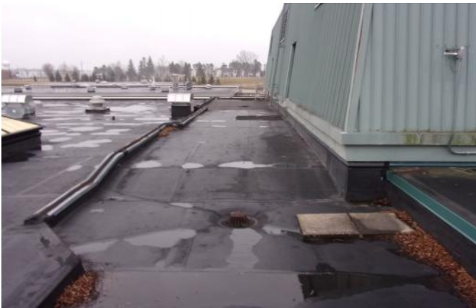
Photo 23 Wylie Elementary School February 2023
