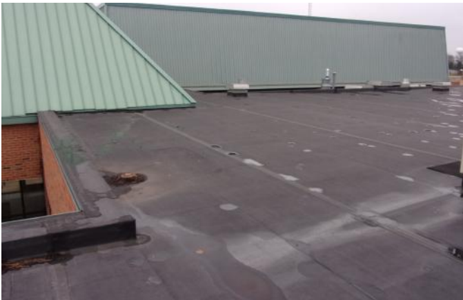
Photo 26 Wylie Elementary School February 2023
