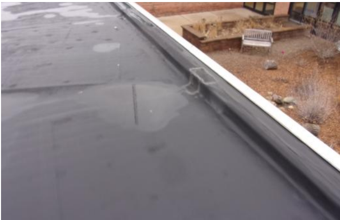
Photo 10 Wylie Elementary School February 2023
