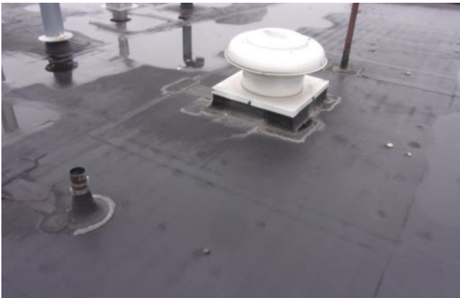
Photo 11 Wylie Elementary School February 2023
