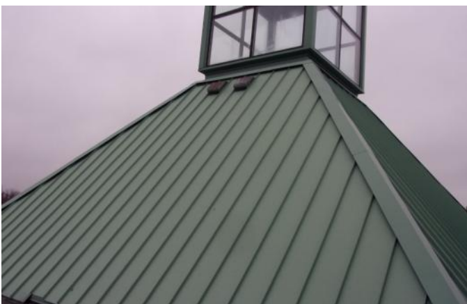
Photo 28 Wylie Elementary School February 2023
