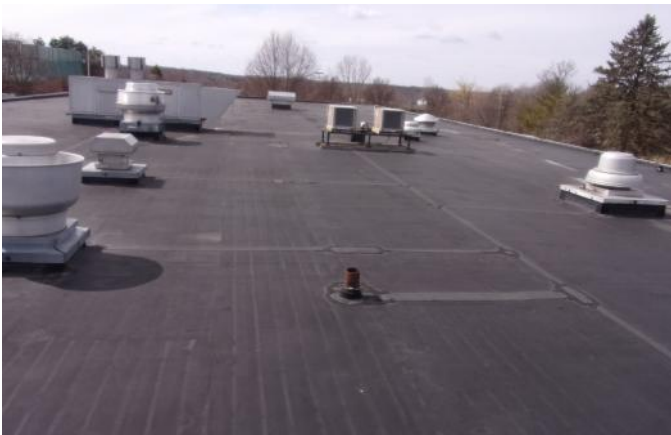
Photo 2 Wylie Elementary School February 2023
