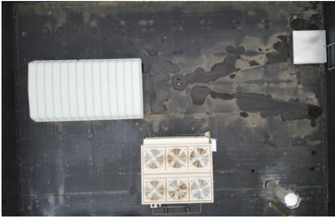
Photo 29 Wylie Elementary School February 2023
