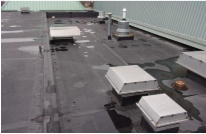
Photo 25 Wylie Elementary School February 2023
