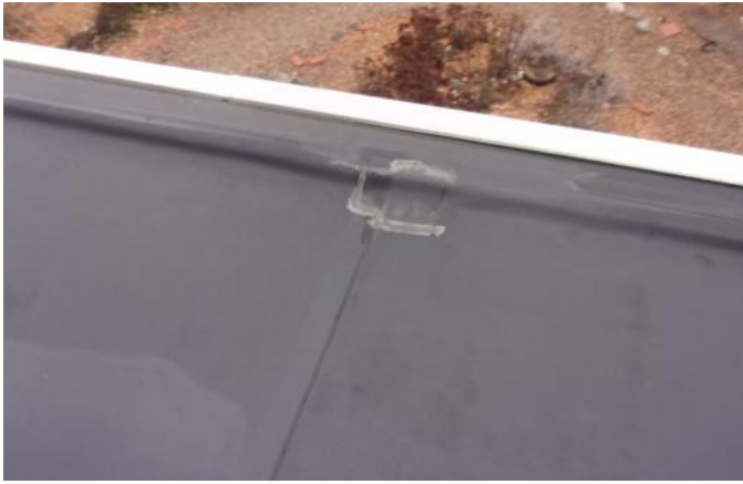
Photo 9 Wylie Elementary School February 2023
