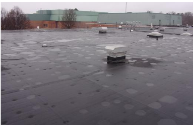
Photo 16 Wylie Elementary School February 2023
