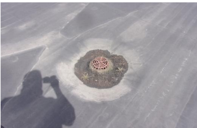
Photo 4 Wylie Elementary School February 2023
