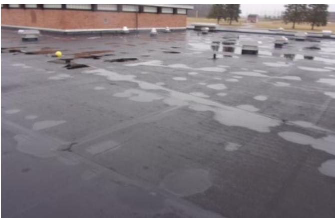
Photo 12 Wylie Elementary School February 2023
