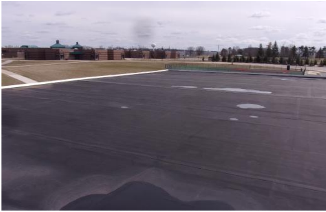
Photo 13 Wylie Elementary School February 2023
