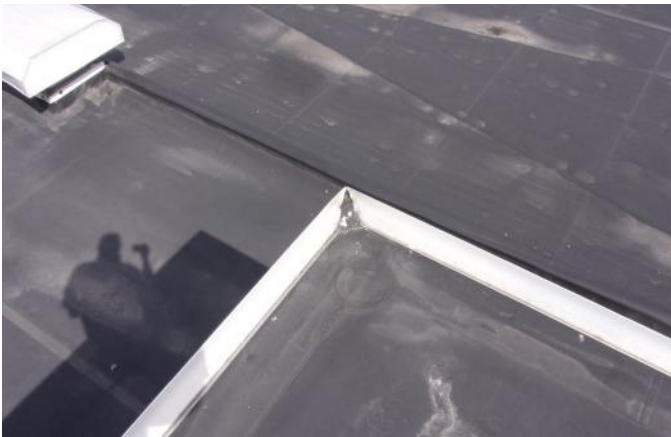
Photo 14 Wylie Elementary School February 2023
