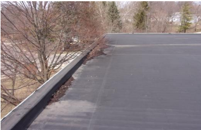
Photo 3 Wylie Elementary School February 2023
