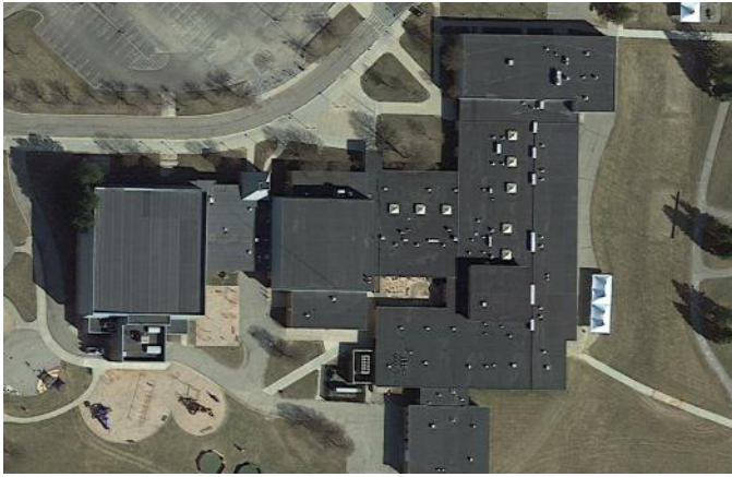
Photo 1 Wylie Elementary School February 2023
