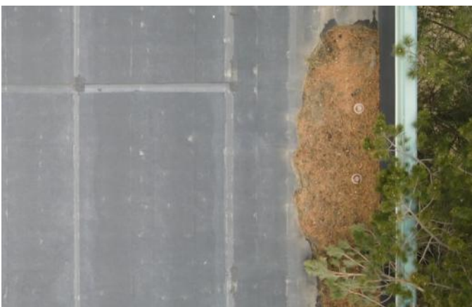
Photo 32 Wylie Elementary School February 2023
