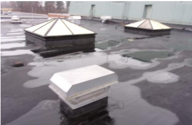
Photo 18 Wylie Elementary School February 2023
