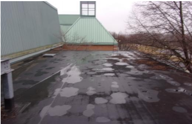
Photo 22 Wylie Elementary School February 2023
