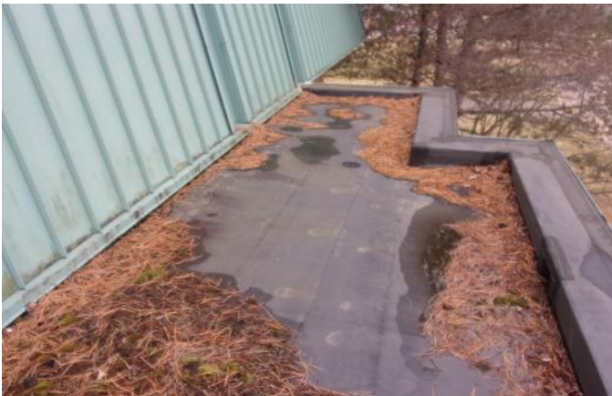
Photo 27 Wylie Elementary School February 2023
