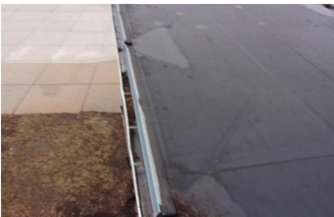
Photo 20 Wylie Elementary School February 2023
