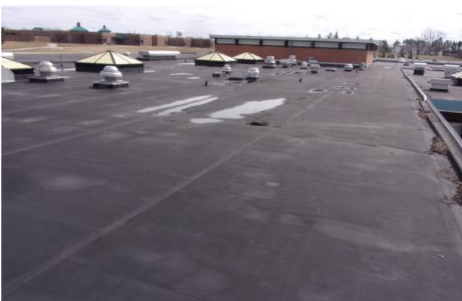
Photo 8 Wylie Elementary School February 2023 Area D: Overview
