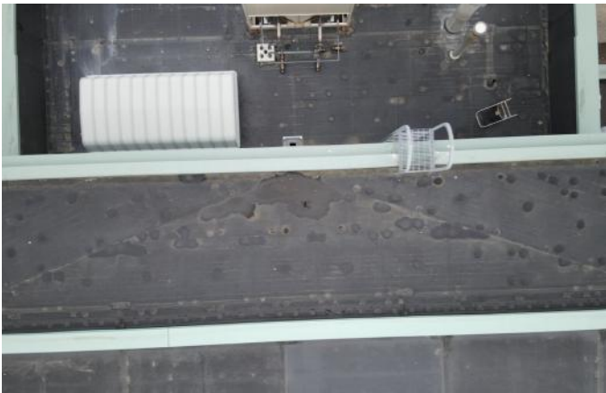
Photo 30 Wylie Elementary School February 2023
